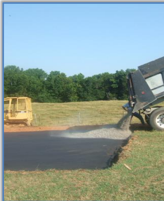
Figure 6.2.a. Constructing heavy use area pads for cattle feeding or watering areas can reduce erosion and sediment loads in the watershed.
