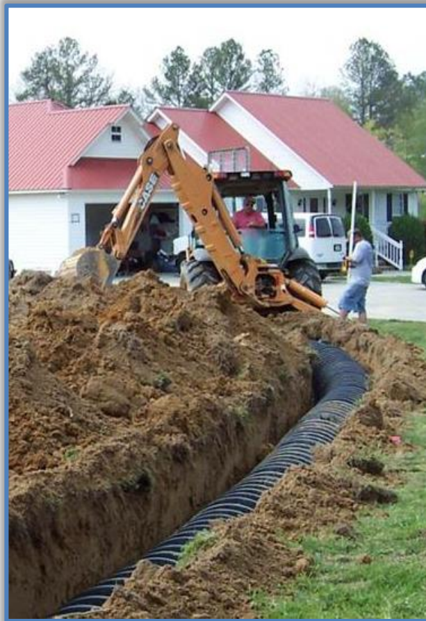
Figure 6.2.b. A septic system repair can reduce the fecal coliform load in streams. A cost-share program can help incentivize costly repairs.
