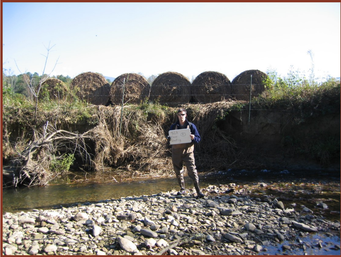
Figure 3.2.c. The above photo is a picture from the Google Earth interactive map documenting a lack of riparian buffer and a vertical, continuously eroding streambank along Holly Creek. Vertical, earthen streambanks tend to slough off massive amounts of sediment into streams making life difficult for sensitive aquatic organisms downstream.
