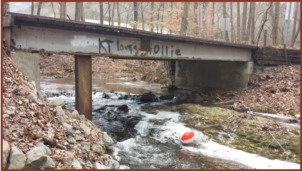
Figure 3.3.h. The bridge that crosses Goldmine Branch/Rock Creek upstream.
