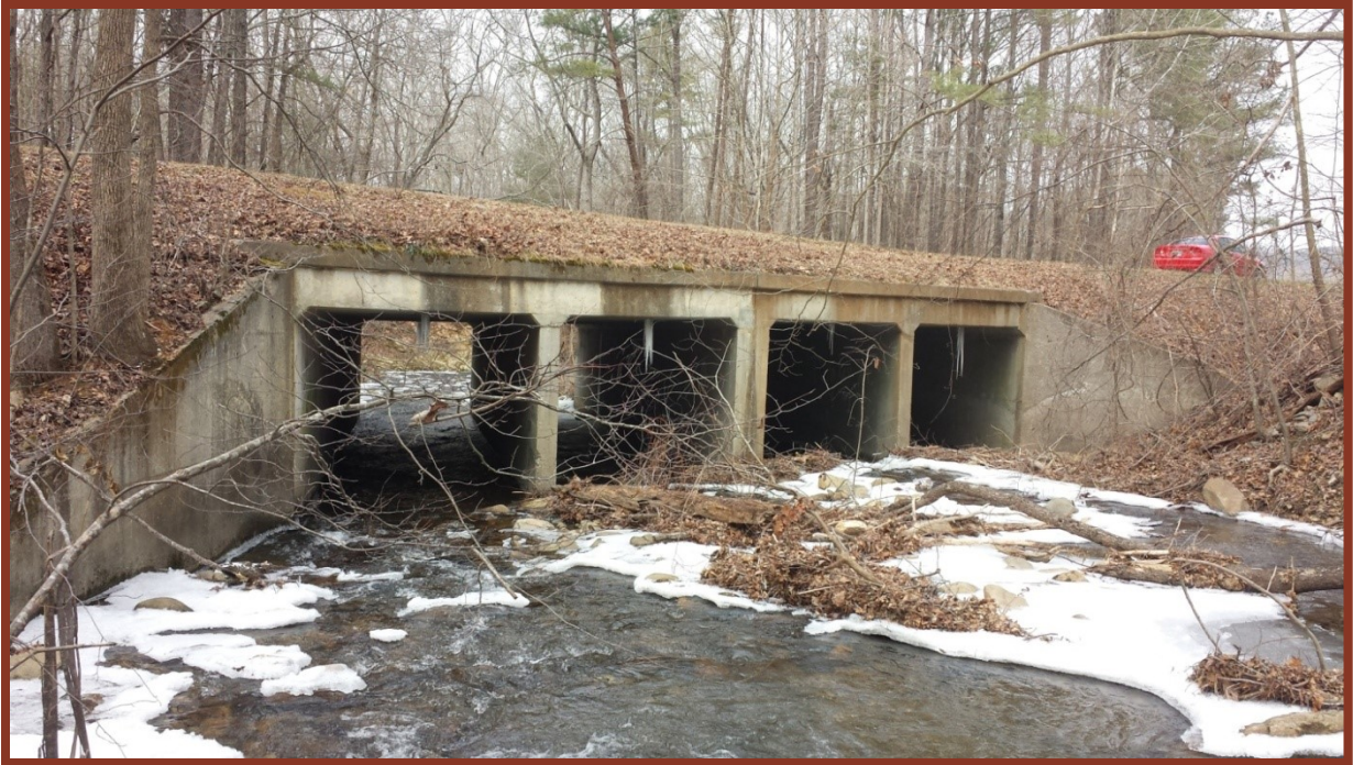
Figure 3.3.c. A photograph of the box culvert that spans Mill Creek on Holly Creek-Cool Springs Road. The structure is the least ideal along Mill Creek, but does appear likely to allow fish passage during most hydrological conditions.
