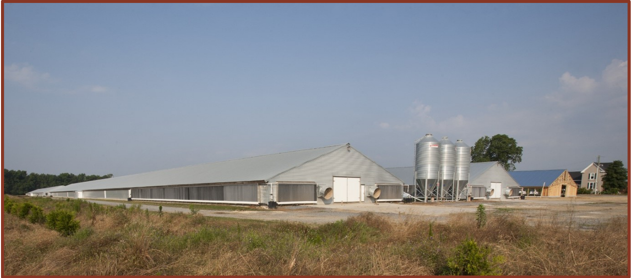
Figure 4.2.a. There are many poultry operations within the Holly Creek Watershed. None, however, exceed the capacity threshold that requires NPDES permits.
