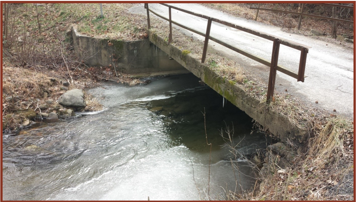
Figure 3.3.d. The free span bridge that spans Mill Creek on Hassler's Mill Road.
