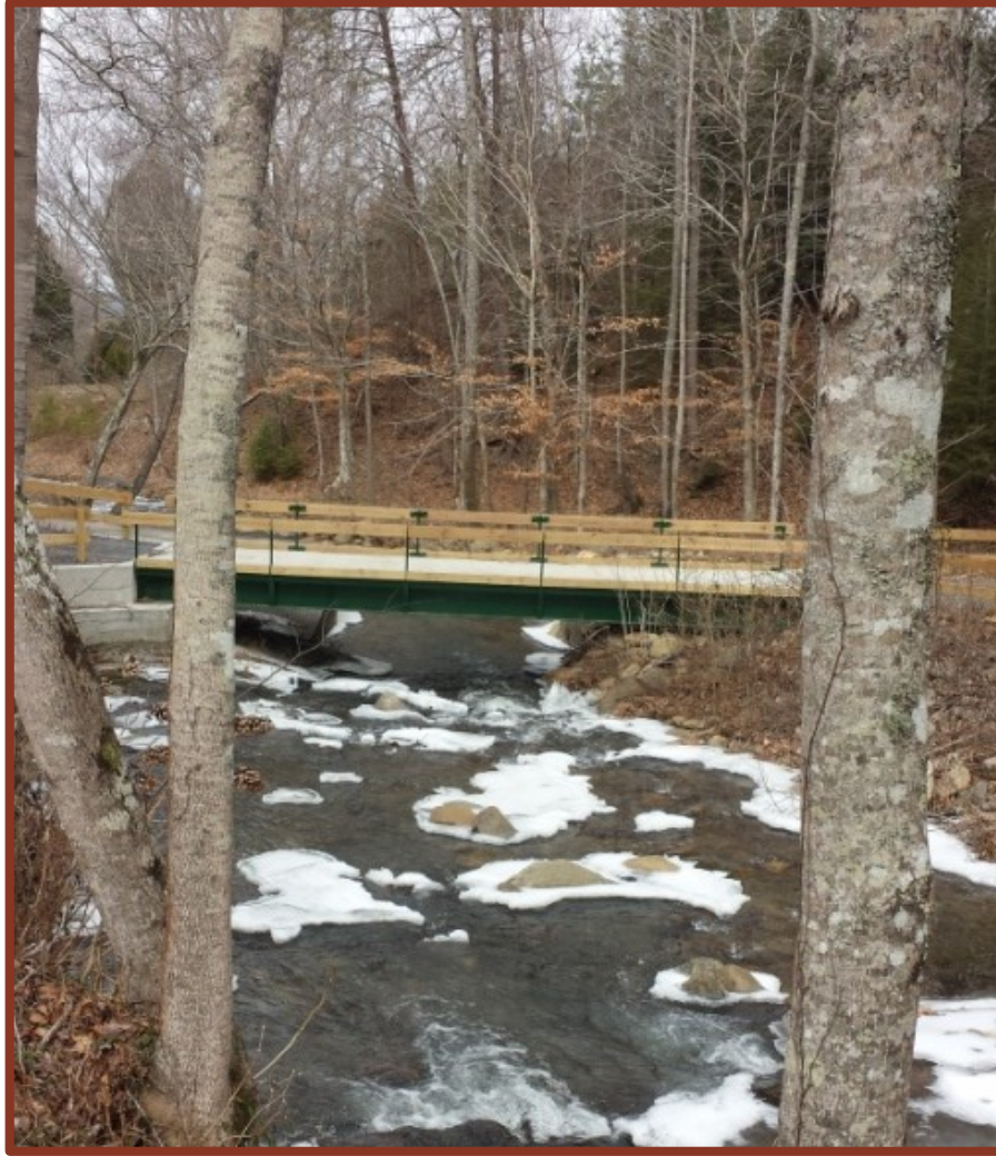
Figure 3.3.e. The free span bridge that spans Mill Creek on a private drive off of Clinton Lunsford Road.
