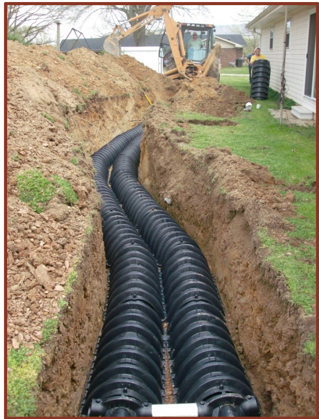
Figure 6.2.b. A septic system repair can reduce the fecal coliform load in streams. A cost-share program can help incentivize costly repairs.
