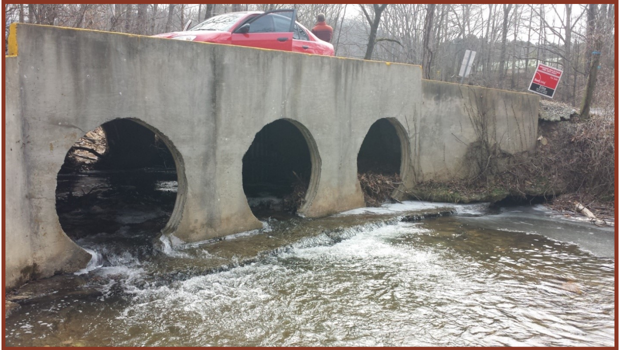
Figure 3.3.f. The concrete culvert that spans Goldmine Branch/Rock Creek on Hensley Road.
