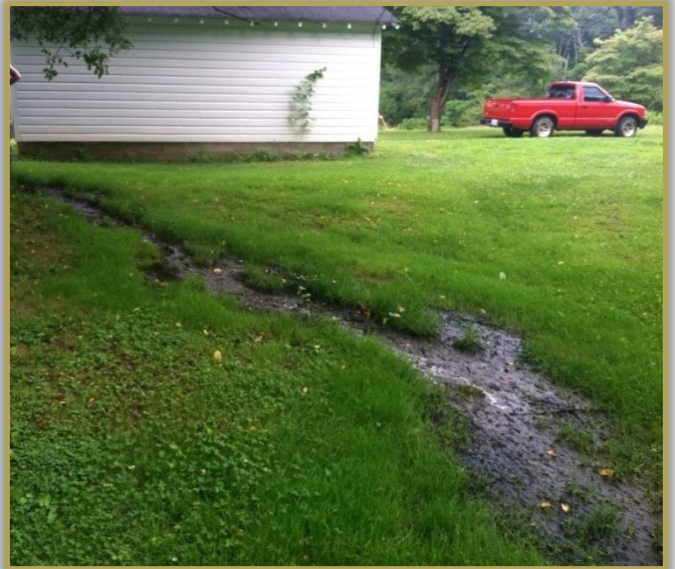
Figure 4.1.c. A failing septic system can introduce pathogens into nearby streams. This system has effluent surfacing in the yard, the vast majority of which drains into a nearby tributary.
