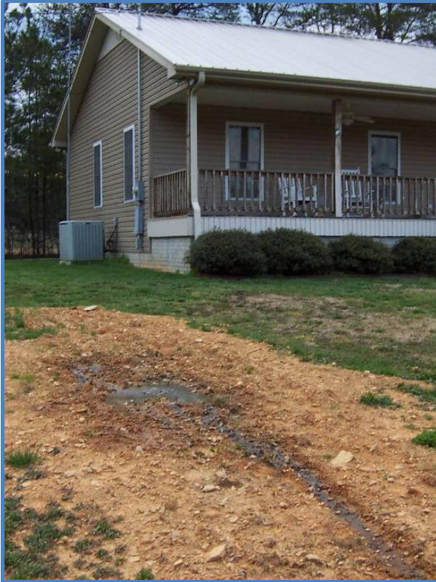
Figure 4.1.c. A failing septic system can introduce pathogens into nearby streams. This system has effluent surfacing in the yard, and drains into a nearby tributary.
