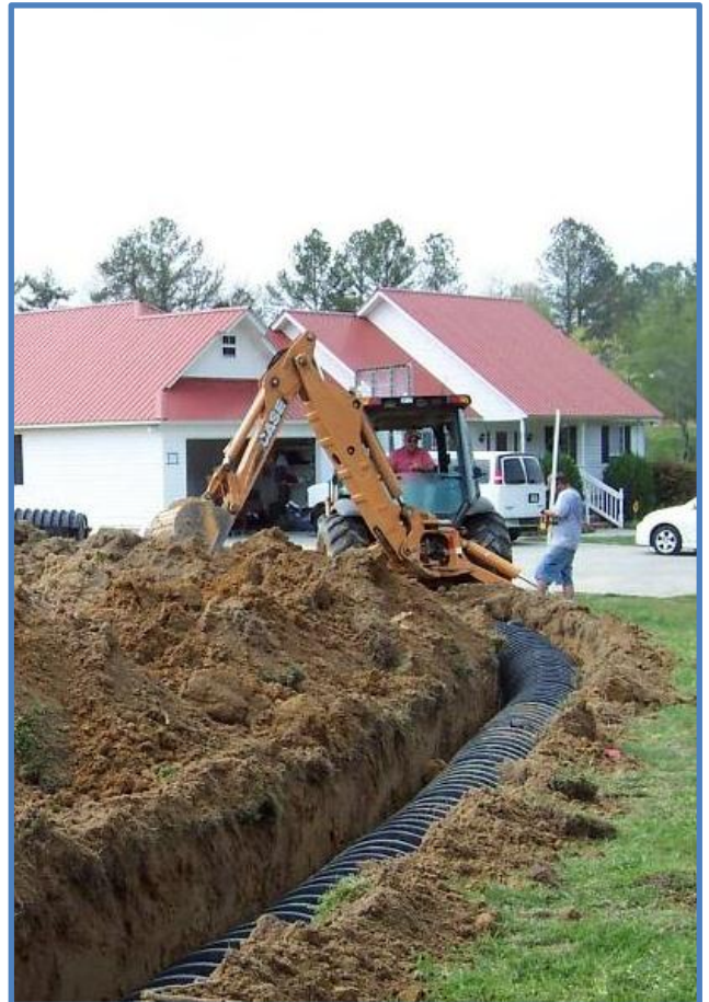
Figure 6.1.b. Septic system field lines are being repaired for this household. There are permitting requirements for repairs in the watershed.
