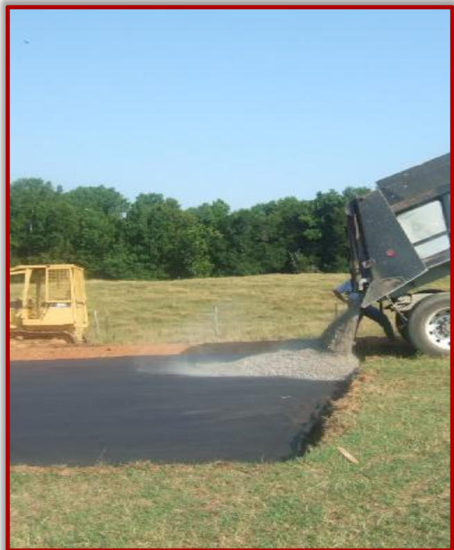
Figure 6.2.a. Constructing heavy use area pads for cattle feeding or watering areas can reduce erosion and sediment loads in the watershed.
